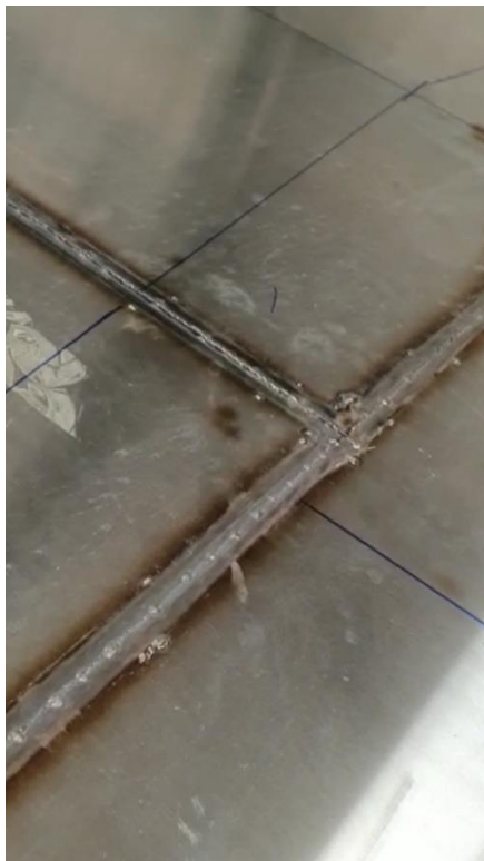
Seam Welded Grinding from sheet surface
